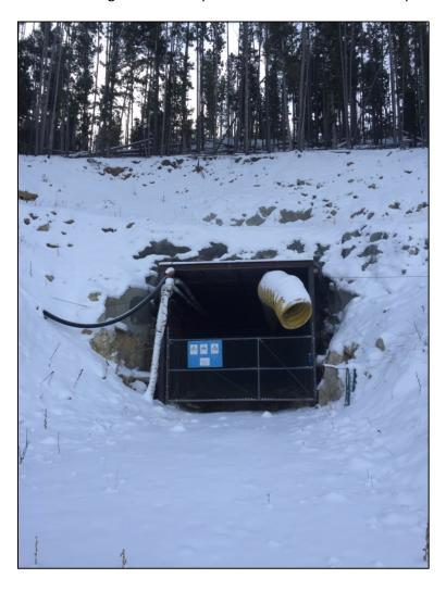
**Inside Elkhorn:** Photo gives the scope of the main access ramp which is a 14' x 14' tunnel. The remaining development will extend the ramp another 800' into the ore body. The ramp will also serve as a haul road for 750 tons of ore per day being hauled from the mine by 30 ton underground mine trucks. From there, the ore is carried by highway trucks 38 miles to the Diamond Hill Mill at Montana Tunnels for processing.
